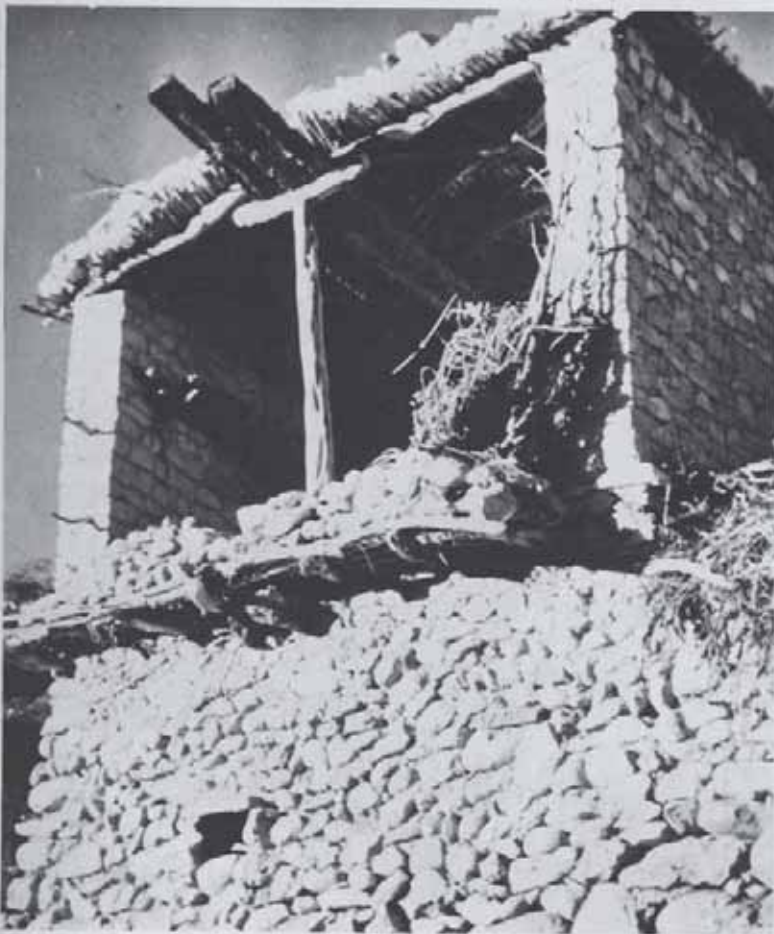
Rhoufi, Aures. Detail showing roof construction reminiscent of tent structure.
