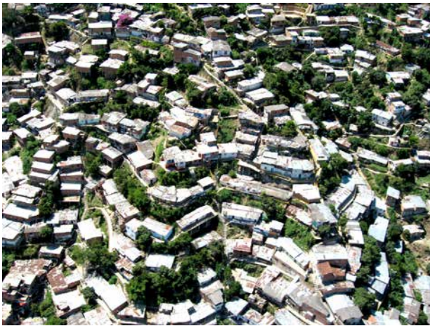
Aerial view of informal settlements in Medellín, Colombia
